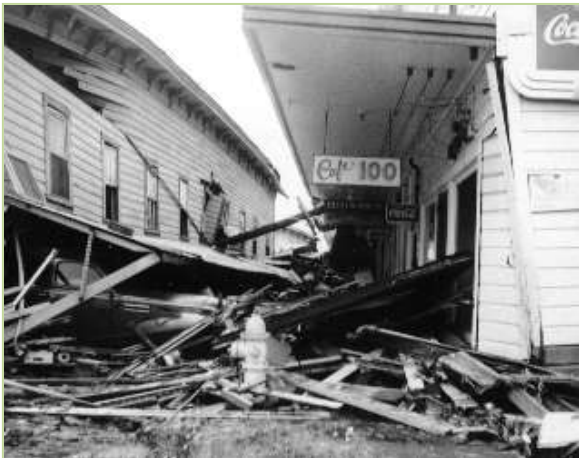
Café 100 damaged after the 1946 tsunami.
